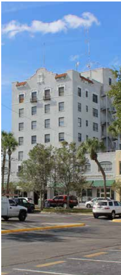
The Sovereign Building in Midtown boasts leaseable office space in a historic building
