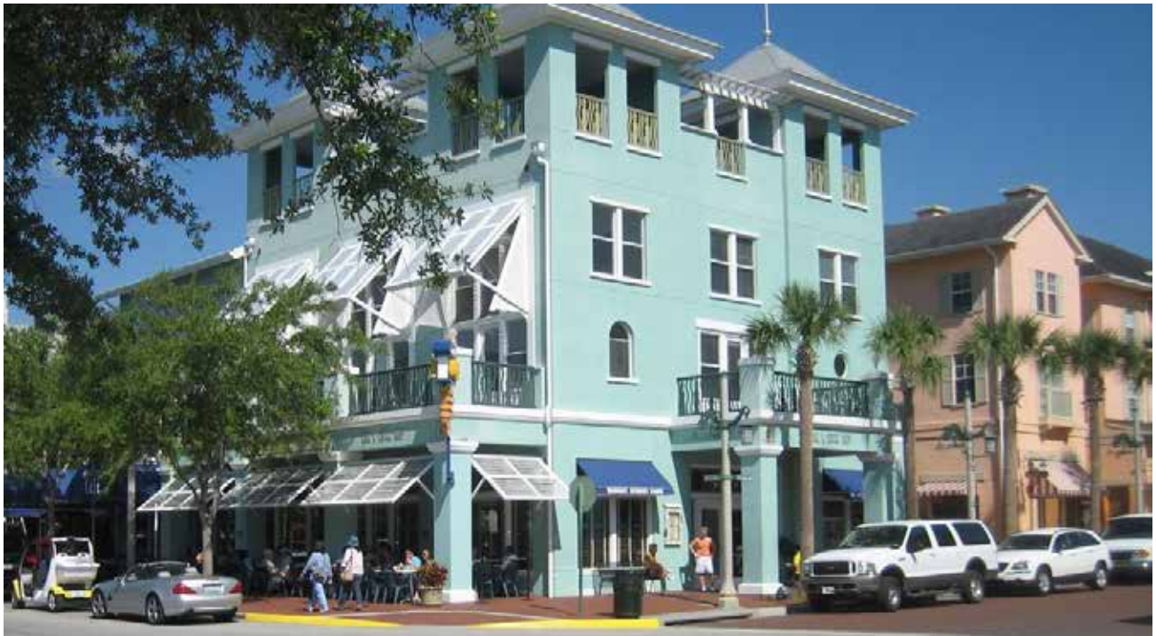
Zoning in Downtown and Midtown supports opportunities for mixed-use development resulting in a variety of land uses and building forms.
